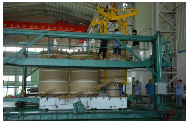
Assemble lifting platform
